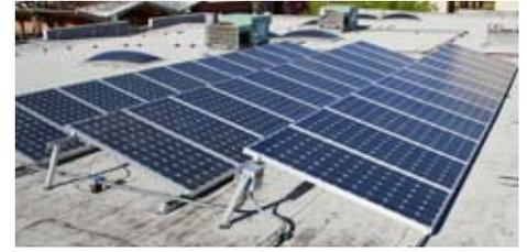
SWEC's rooftop photovoltaic array consists of 33 panels in three rows. Photo Ken Stinnett.
